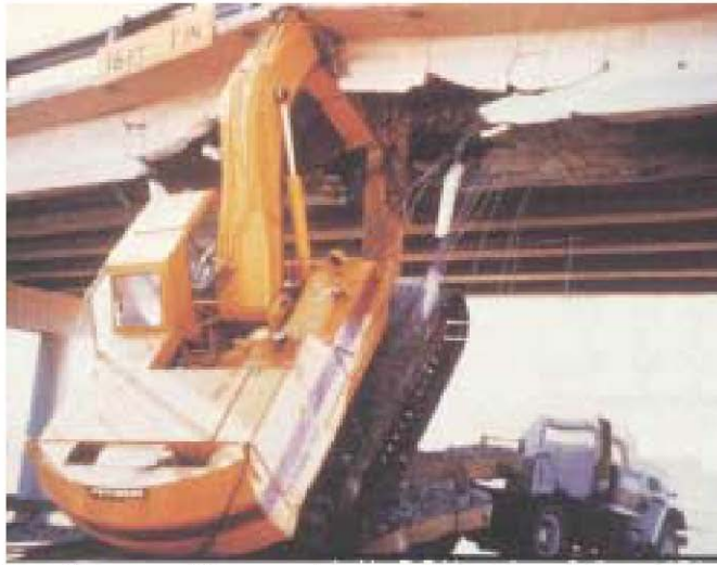
Figure 1: Accident caused by inaccurate bridge/vehicle clearance information
